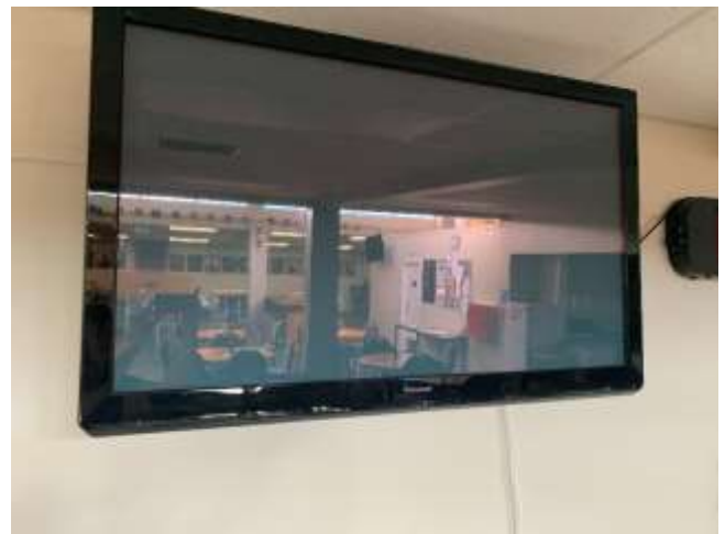
Panasonic Television 55 Inch Wall Mounted Bracket Wiring & No Remote
